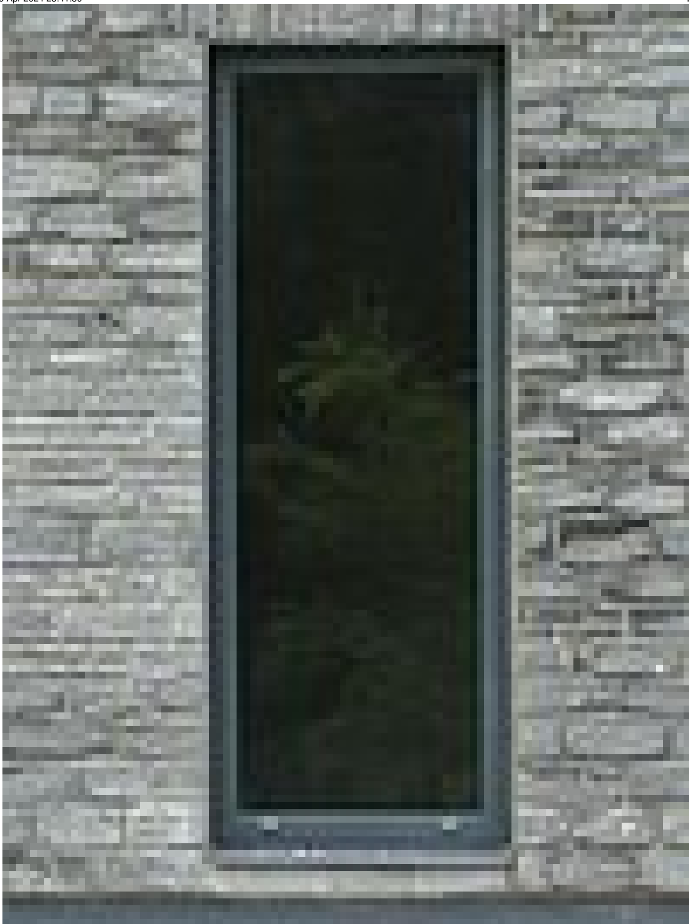
Window with thermo glass and hinged frame F2
