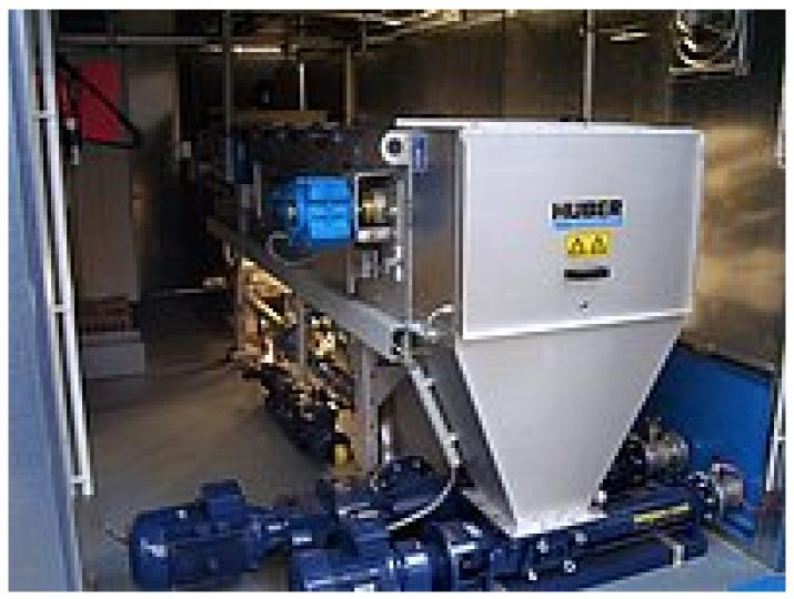
Belt thickener for highly efficient sludge thickening
