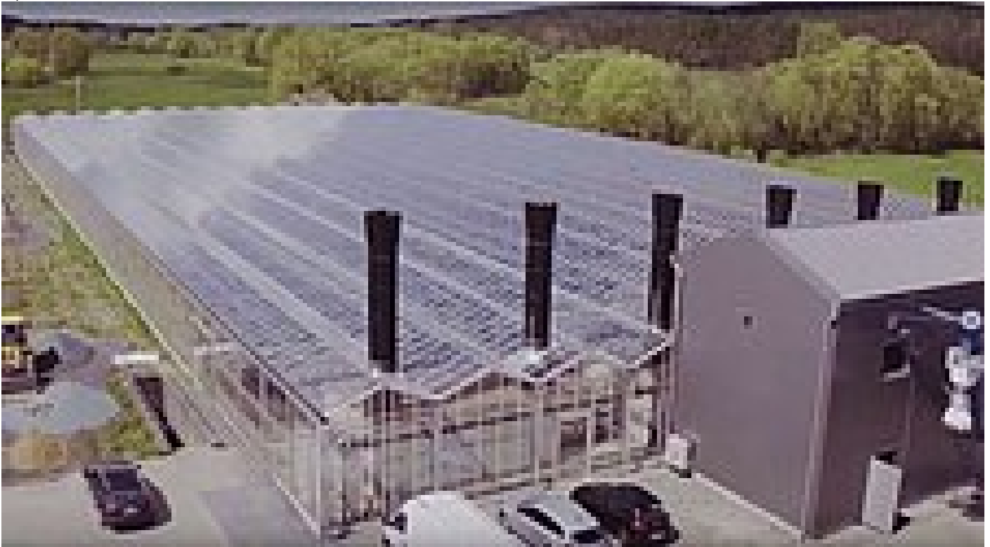
Aerial photo of the sludge drying plant in Bayreuth
