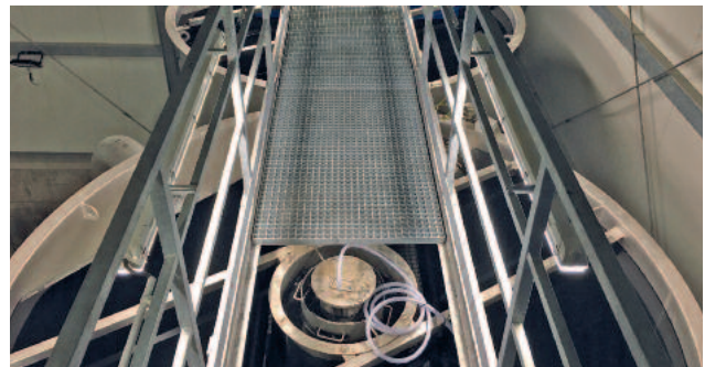
Combination of disc filtration with activated carbon filtration (GAK) and downstream UV disinfection (5th treatment stage)
