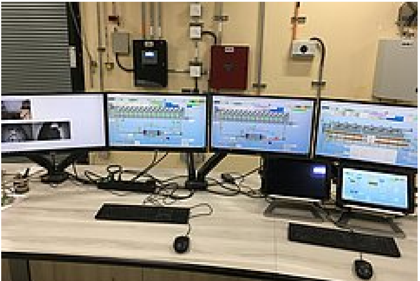
Control system for the drying plant
