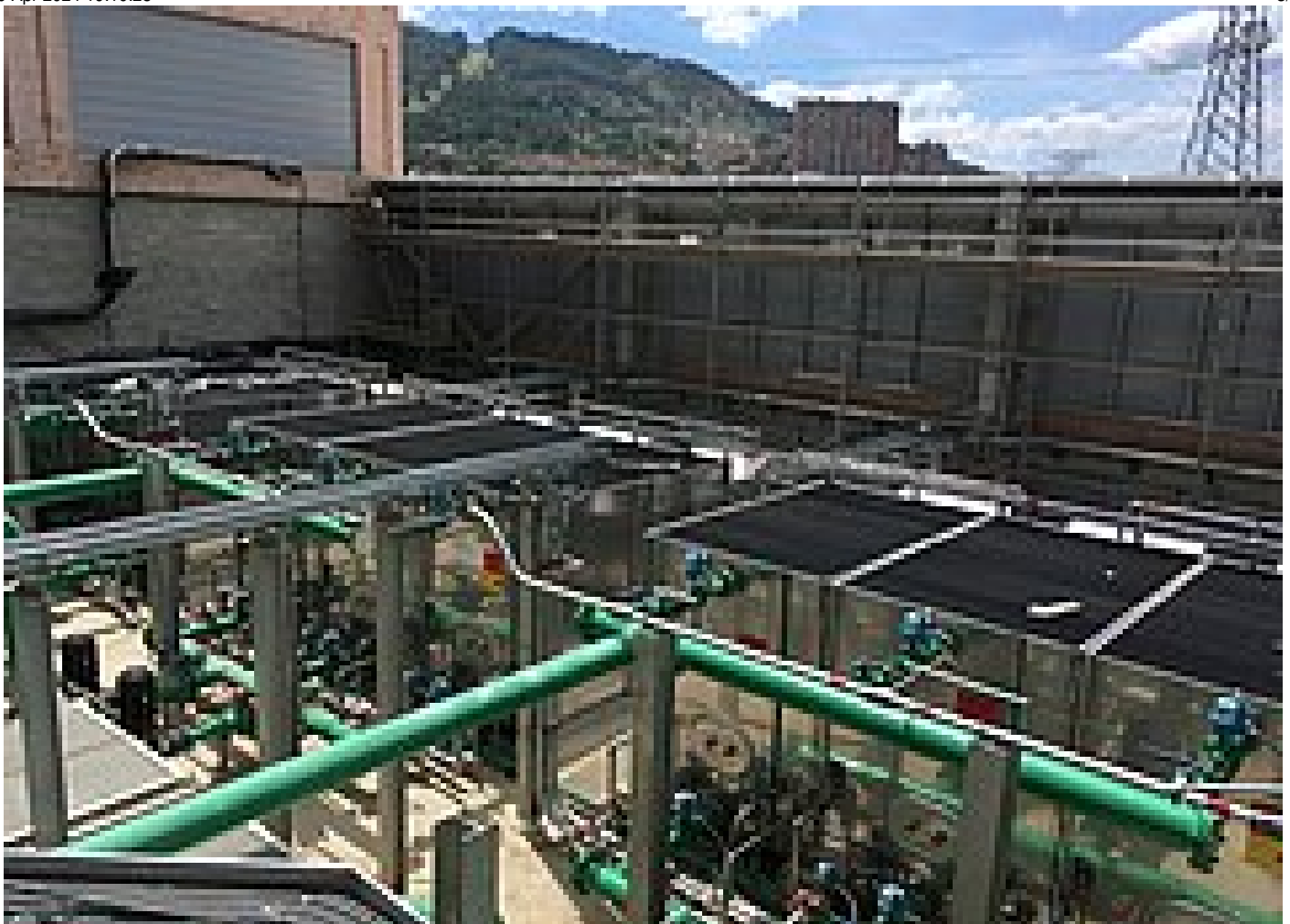
Cooling towers and exhaust air treatment
