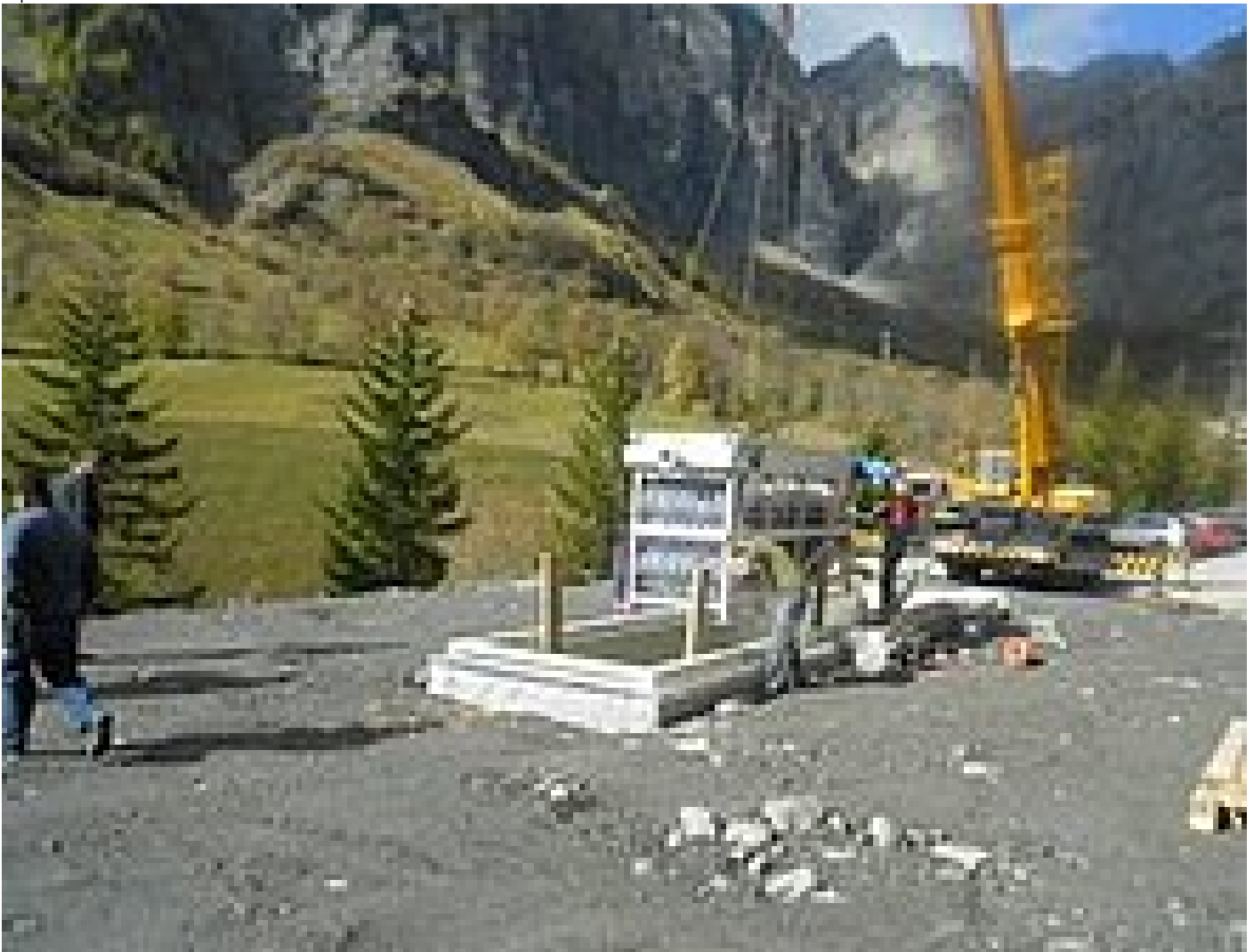
HUBER RoWin Heat Exchanger (tank version) during installation
