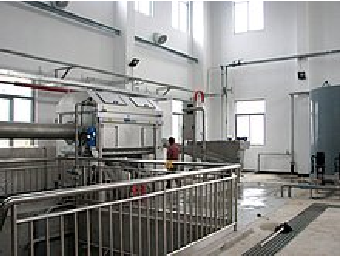
Fig. 4: Screening with an ultra-fine RoMesh® Rotary Drum Screen
