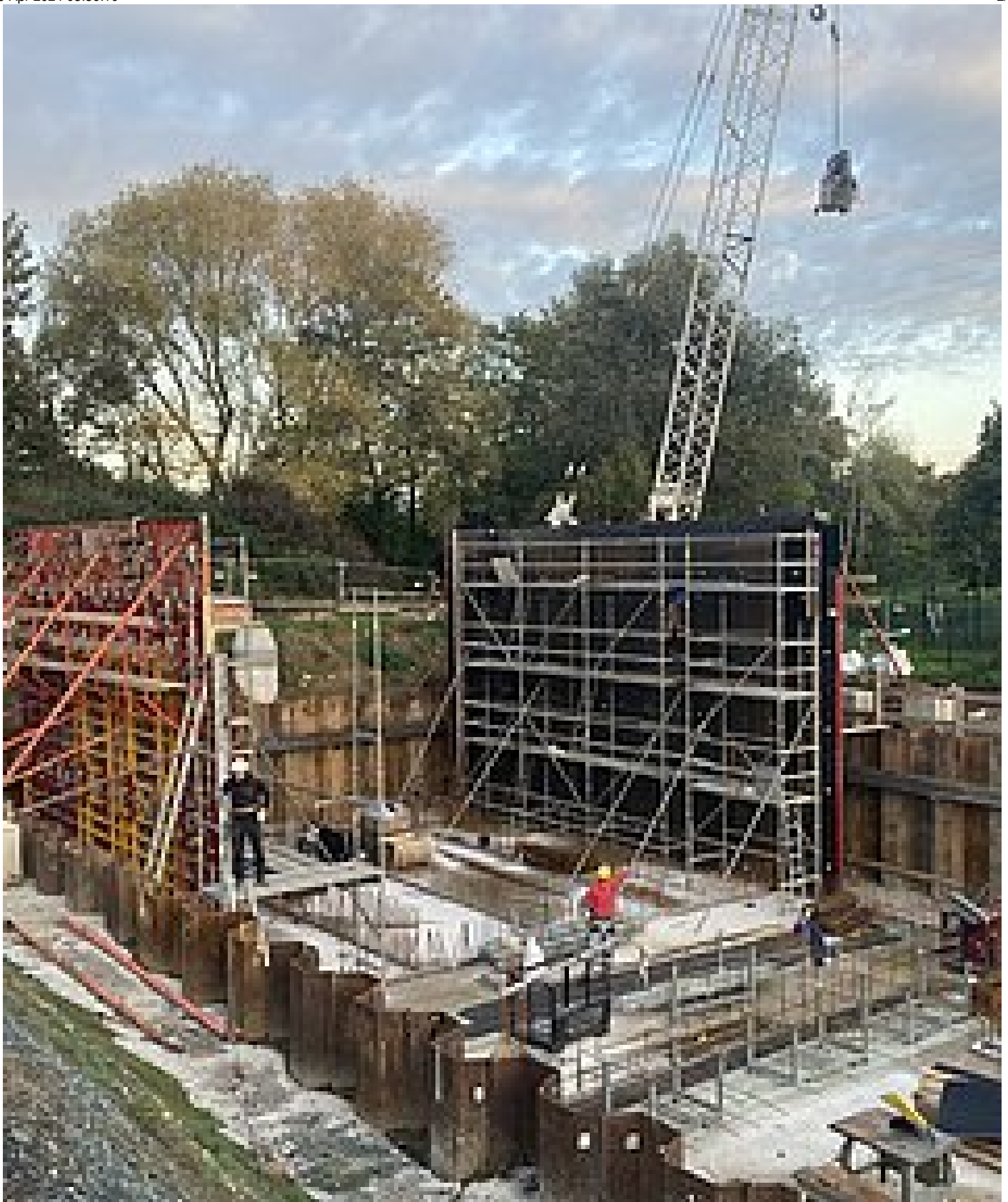
Construction of the activated carbon filter stage in Bickenbach is progressing. (Photo: Jörg Stanzel, Wastewater Association Bickenbach)
