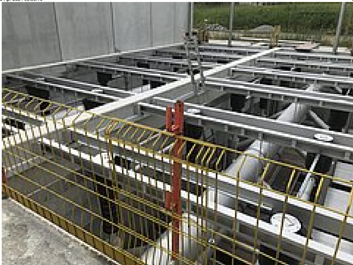
In Uhdingen, the 24 HUBER Activated Carbon Filter CONTIFLOW® GAK units were already installed in summer.
