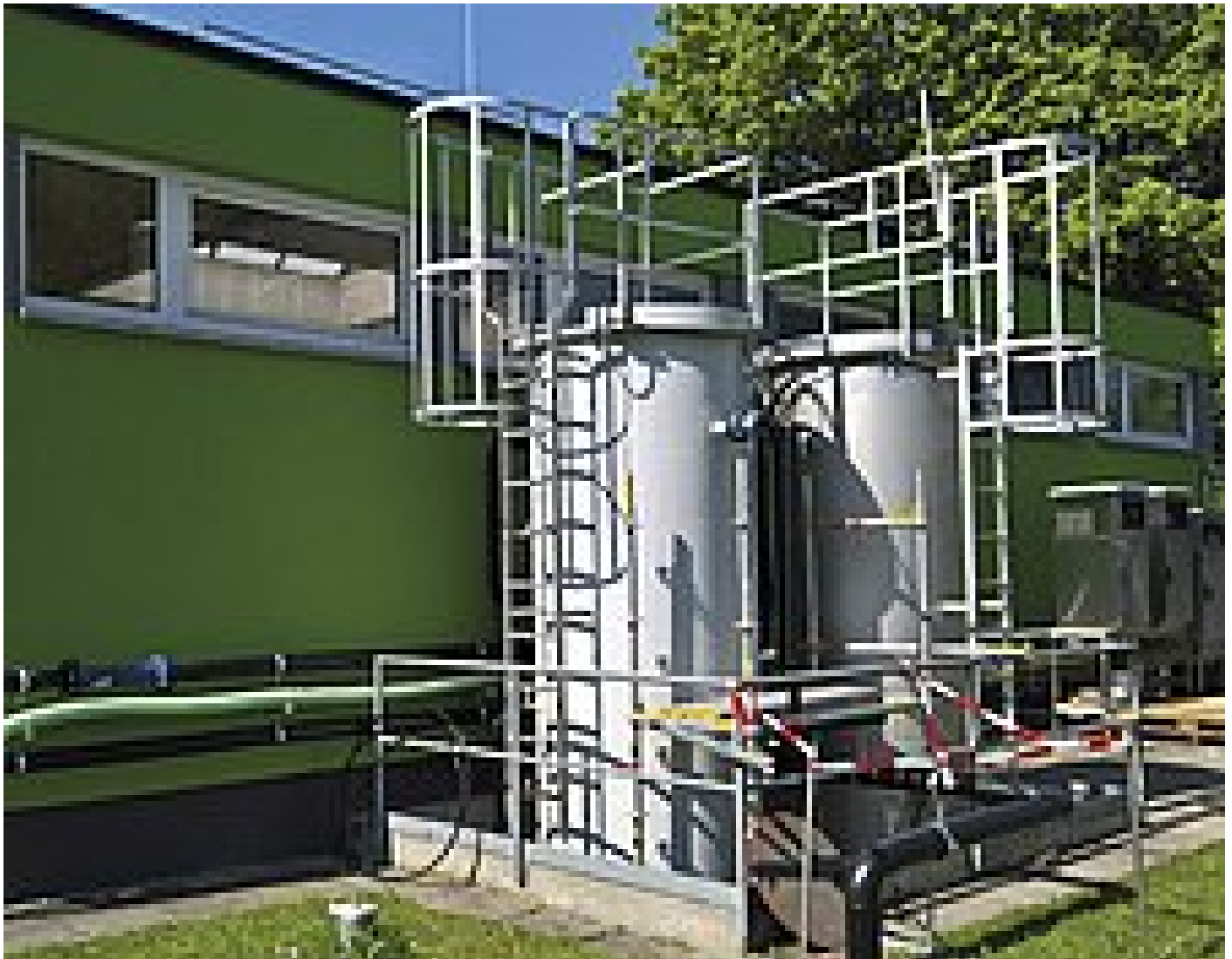
Active carbon filtration on the central wastewater treatment plant at Boehringer Ingelheim
