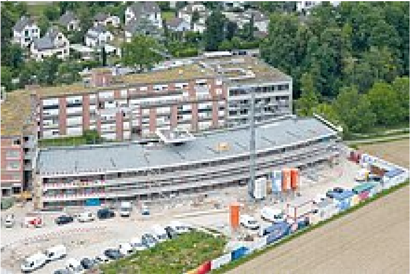
New retirement and nursing home Hofmatt in Münchenstein
