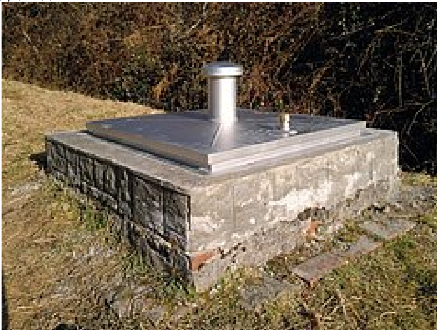
Weatherproof manhole cover
