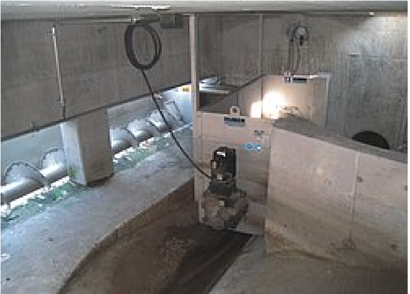
Stormwater overflow tank at Kappern: Storm Screen RoK1 on the left, Storm Screen RoK2 in the middle on top of the sewer towards the WWTP
