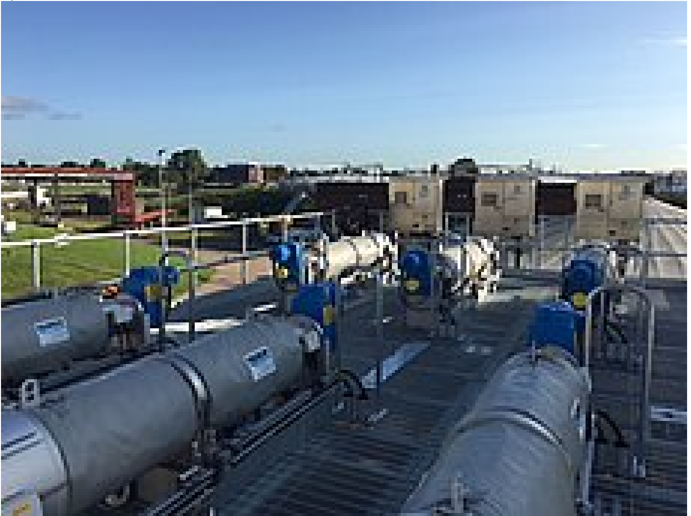
Minworth STW STRAINPRESS® Installation
