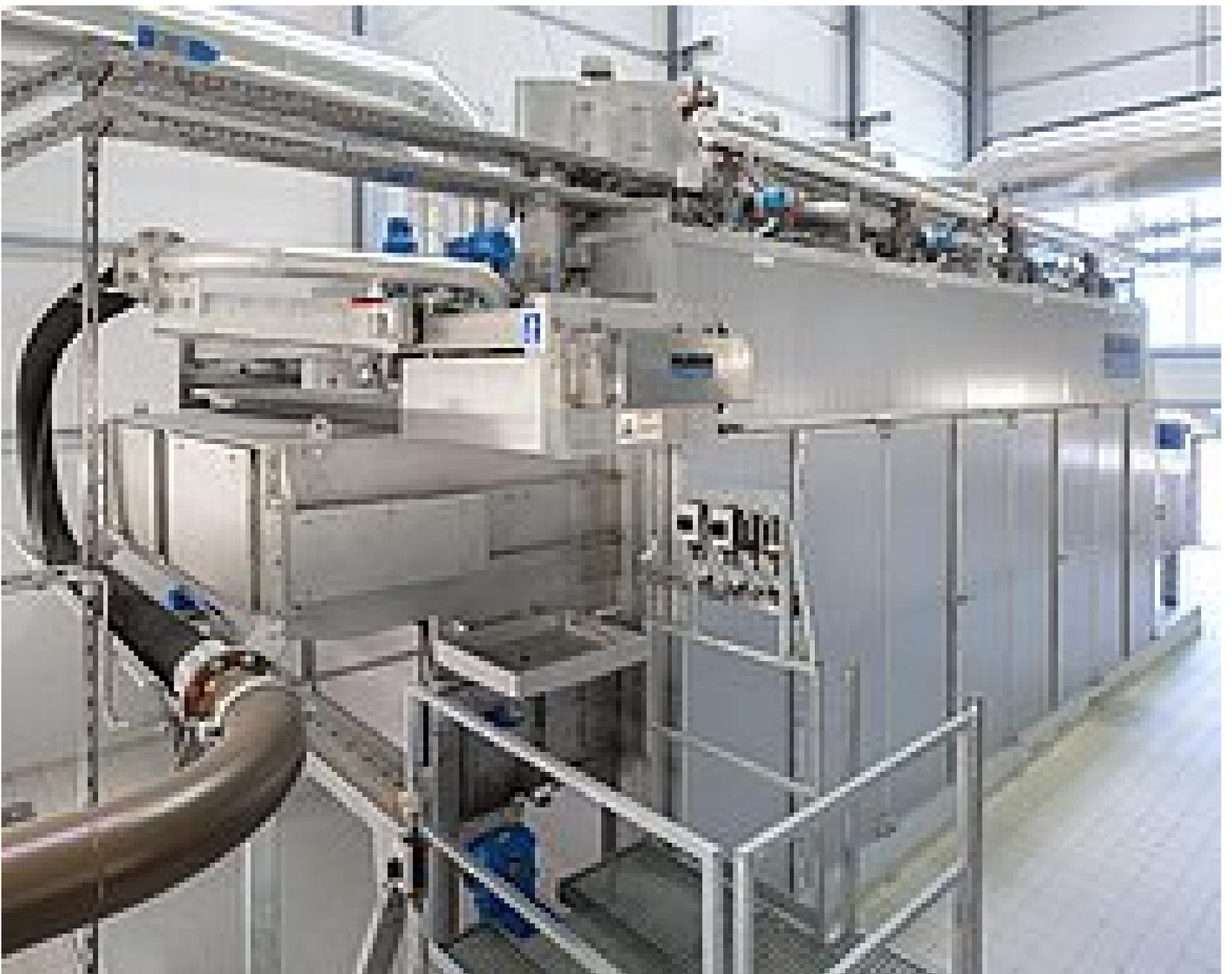
Fig. 3: HUBER Belt Dryer BT 8, rear view
